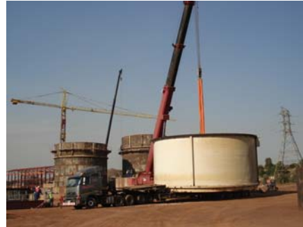
ERECTION OF TANKS AT WERGO
