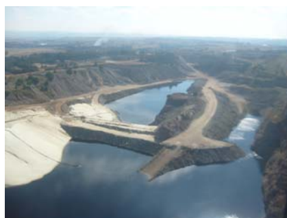
WEST WITS PIT DIVISION WALL
